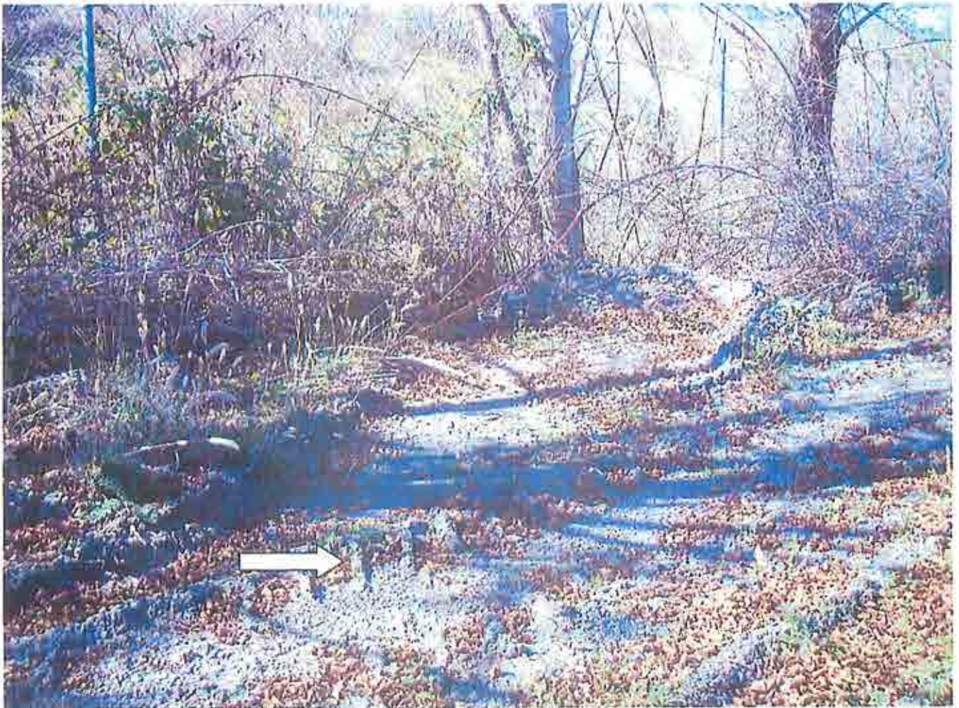
Photograph 5. Equipment tracks (arrow) left from apparent breaching of straw wattles. Straw wattles were intact in other areas of the site, however, at this point, they appeared to have been removed and runoff directed toward the tributary to the Mad River.
