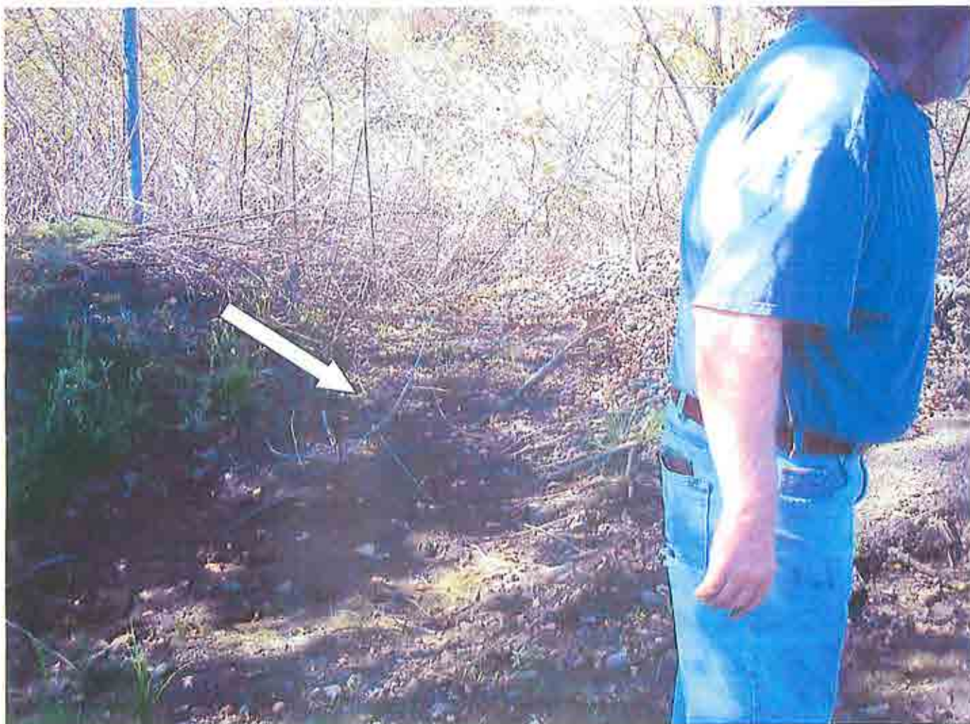
Photograph 4. Area cleared (arrow) by equipment for apparent enhancement of storm water runoff into a tributary leading to the Mad River. The area appeared to have previously had straw wattles installed. However, a low area was created with equipment to apparently allow water to flow offsite and into the tributary to the Mad River.
